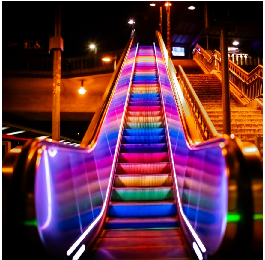
TKE escalator with colourful steps at a railway station in Freiburg, Germany
